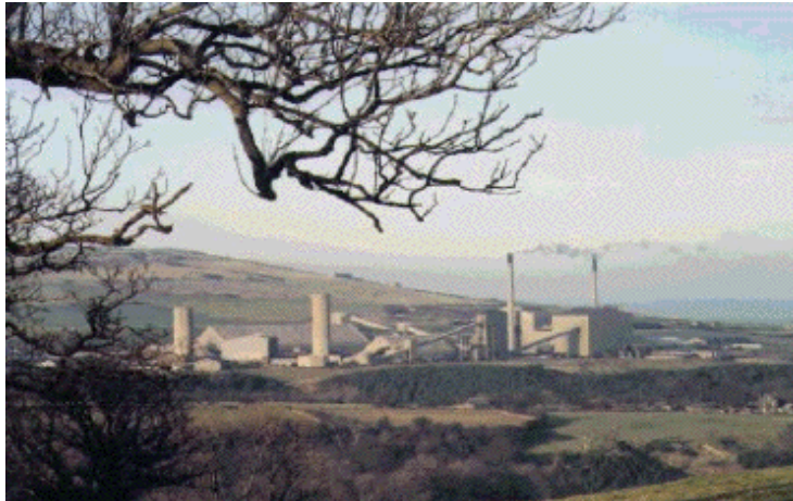
Figure 4: Boulby Mine in Yorkshire.
